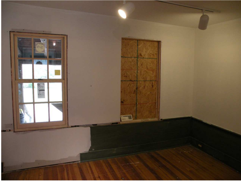
Laurie's work area ready for paint
