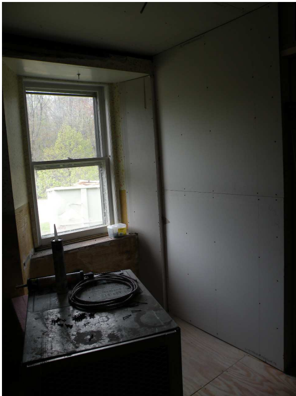
Old bathroom window now part of the new library
