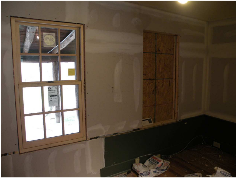
Another view of the new window
