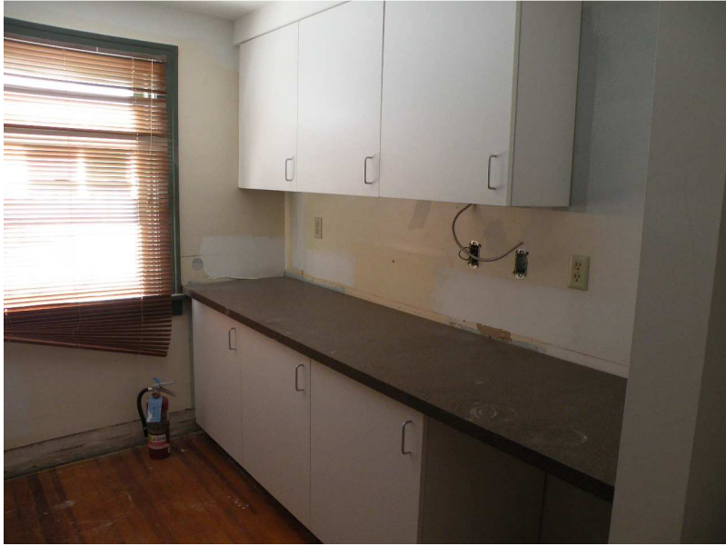
New mail & work area cabinets
