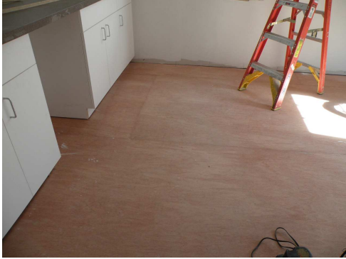
Subfloor in new addition
