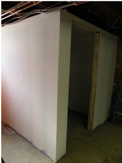
Basement restroom has been primed
