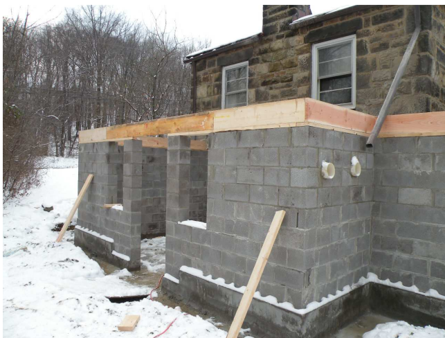
The carpenter's started the framing
