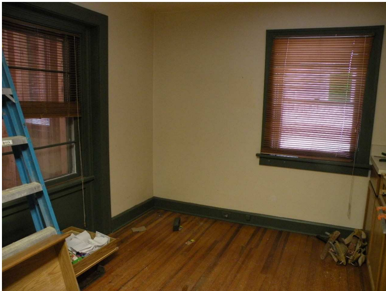
Old kitchen new work area and
