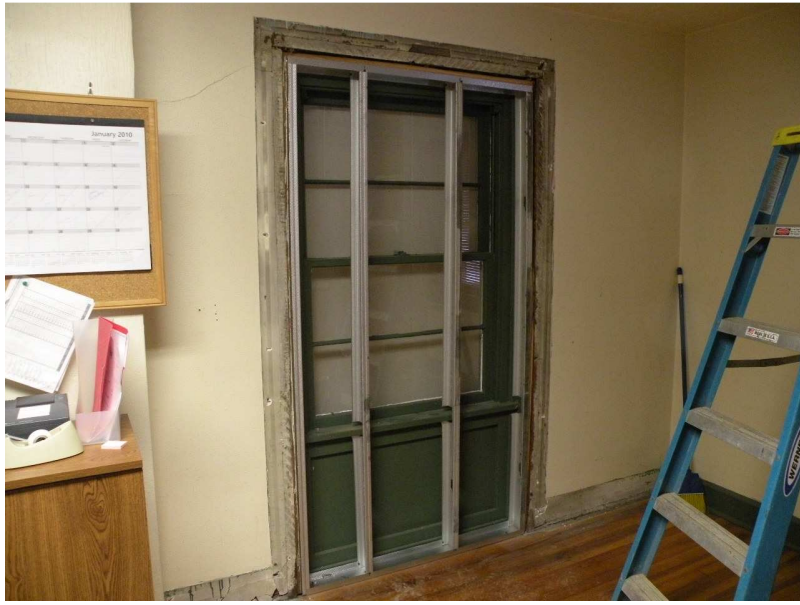
Kitchen window will be a wall
