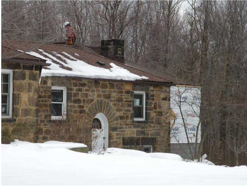
Shingles and roofing finished
